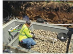
**Eliminite** is a denitrifying septic system developed in Bozeman, Montana. Two 1,500-gallon concrete tanks treat all household wastewater (both blackwater and greywater)
